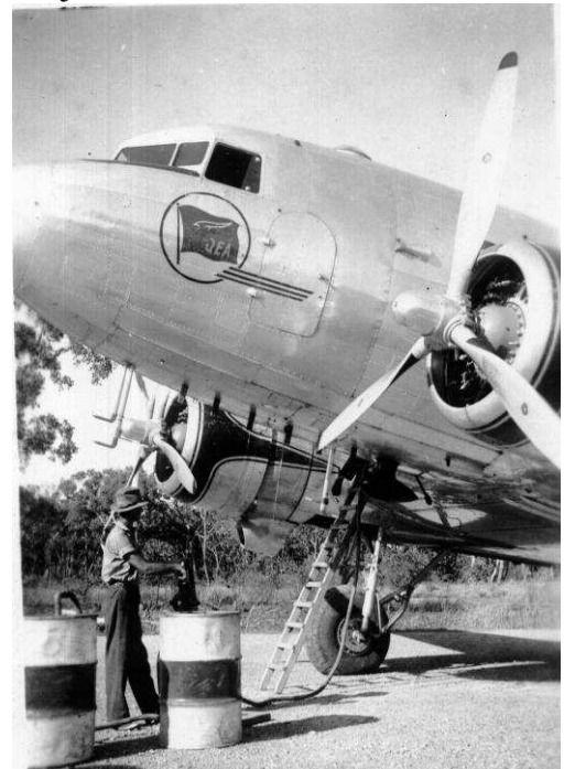
Cooktown Mission Strip 1948 - refuelling the aircraft from a 44 gallon drum with hand pump.
